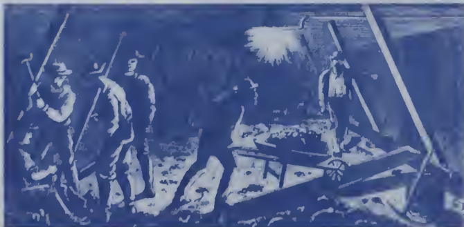
The men in the caisson excavate the rock with chisel and sledge hammer, pick and shovel by the light of a gas flame. Fire was a constant danger in the timber caissons.
